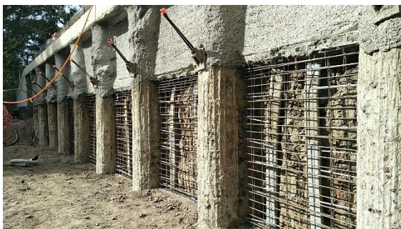
iii. Reinforcement for shotcrete
