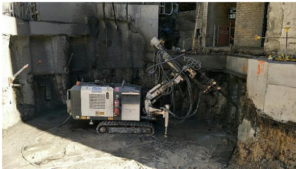
i. Rig drilling for anchors
