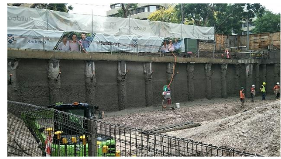
IV. Shotcrete to southern elevation
