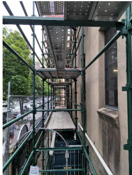
iv. Perimeter Scaffold for Catering
