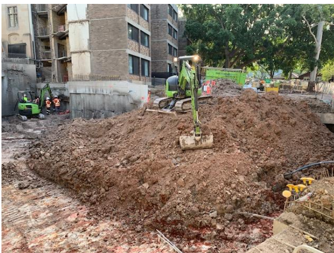
Bulk excavation and loading out
