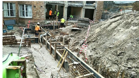
ii. Formwork to capping beam for TRL
