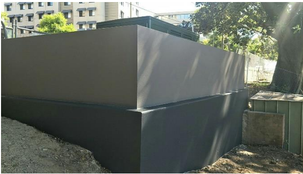
i. Render to Blockwork for Substation
