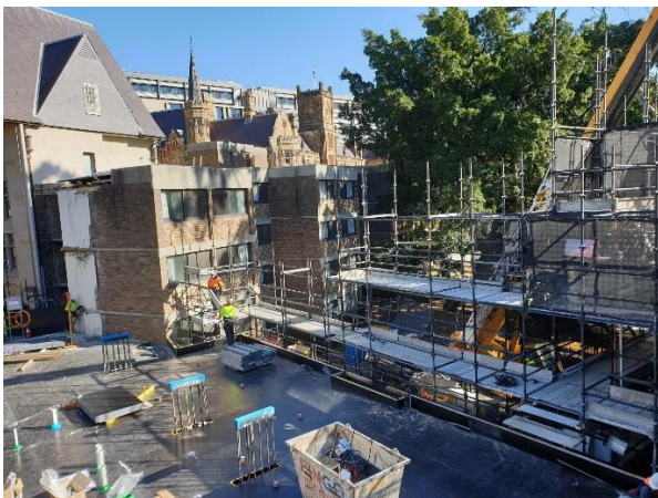
i.Scaffold erection
