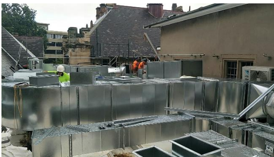
iii. Roof Plant Installation for Catering
