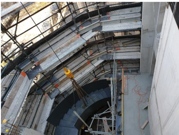
iii. Steel Stair Install
