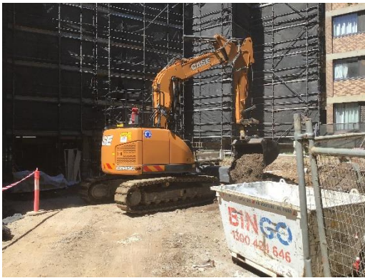
i. OSD tank excavation
