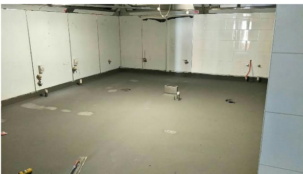
iii. Membrane to kitchen floor
