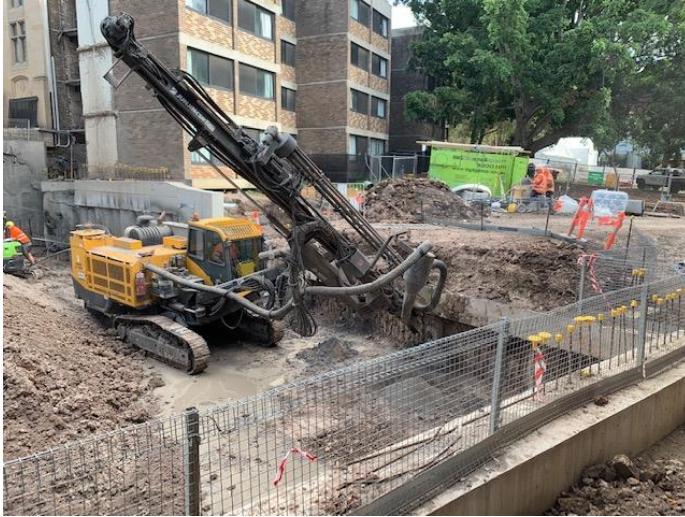
Anchor drilling rig
