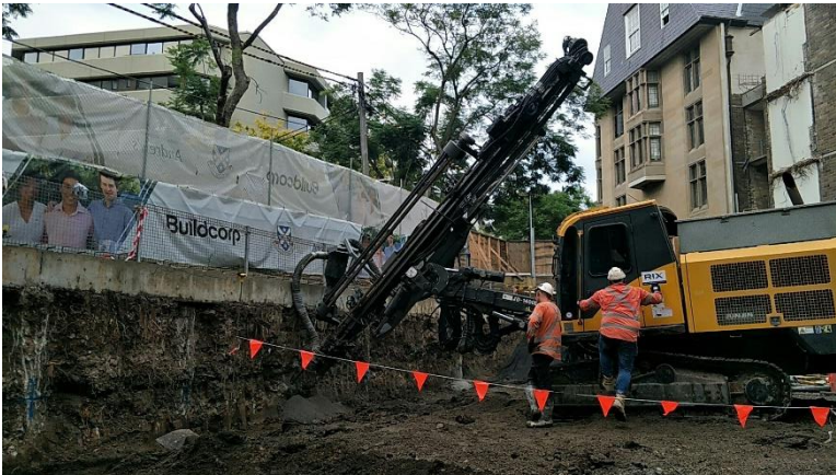
iii. Anchors being drilled
