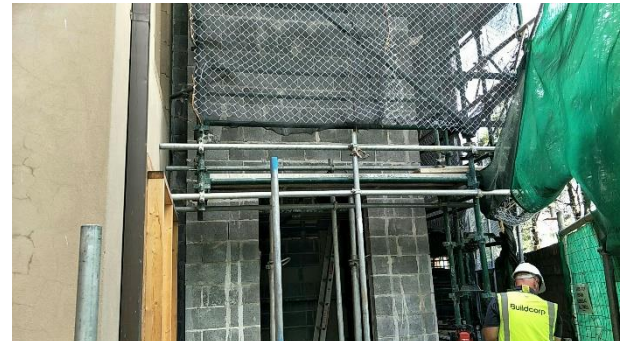
iv. Blockwork lift shaft
