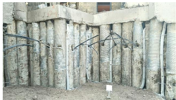
ii. Installation of anchors
