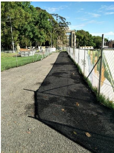
iii. Access road (Sealing Commenced)
