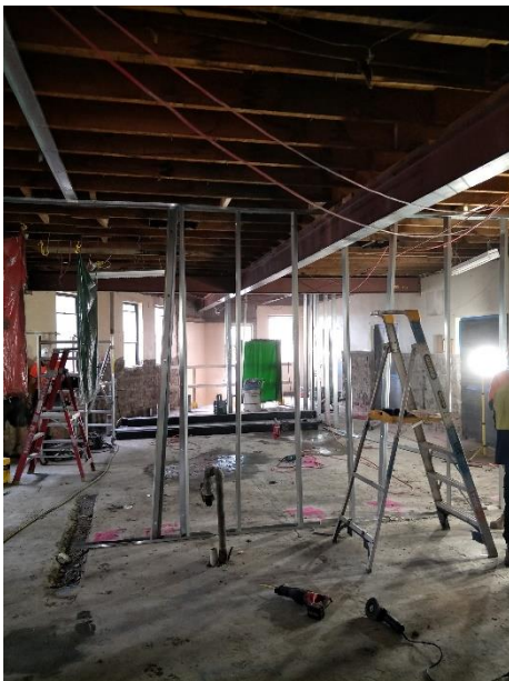
iii. Stud walls to Catering
