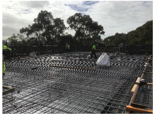
ii. Reinforcement to L7
