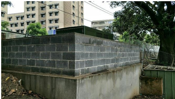
i. Blockwork Wall to Substation
